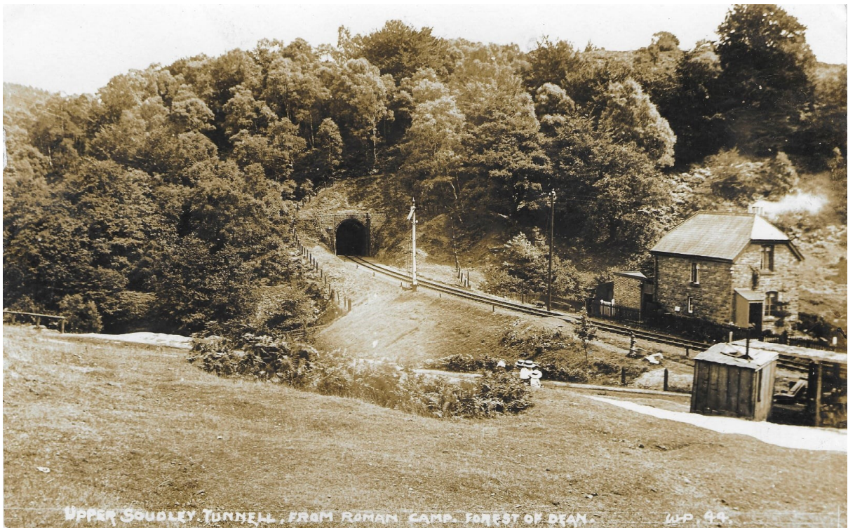
A slightly later photo of the cottage than the one at the start. The cables etc. running down the wall, are now missing.
